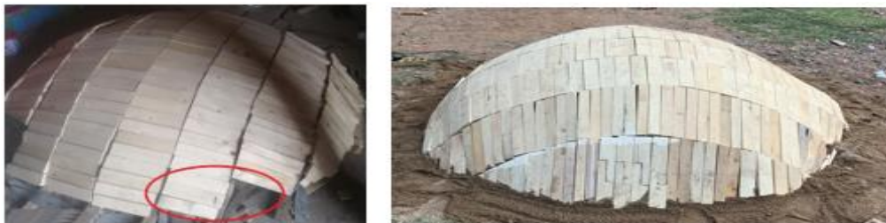
Fig. 7. Formwork membranes in position
