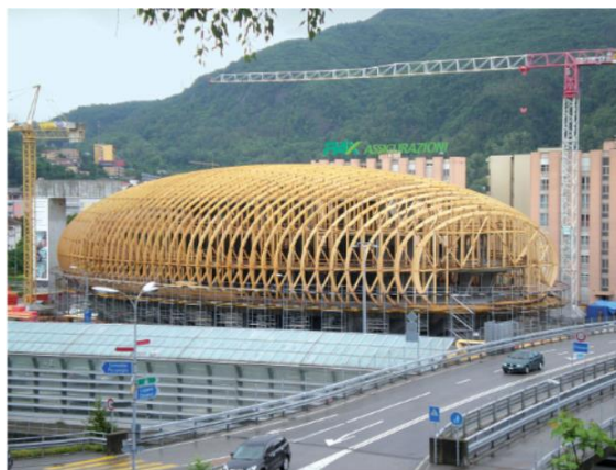
Fig. 1. Wooden Formwork of 93x52 m for shell in Chiasso, Switzerland (Photo credit: Aurelio Muttoni)
