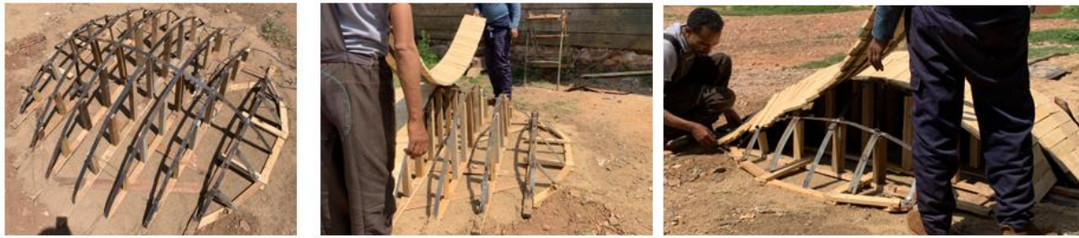
Fig. 6. Formwork supports and membrane laying
